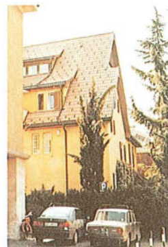
172 Casa via Montello 6 p.ed. 685
