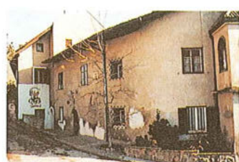
90 Maso - Via Rivellone 2/4 - p.ed. 213 - 214
