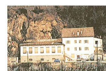
155 Maso - via Rafenstein 7 - p.ed. 142/2
