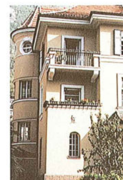
106 Villa Oberrauch - via Cavour 21 p.ed. 901 - p.f. 191/11
