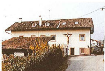
139 Maso - via Eisenkeller 7 - p.ed. 297
