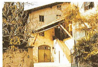
92 Maso - via Rivellone 9/9a - p.ed. 208
