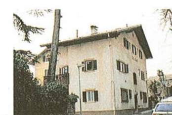
156 Maso - via Rafenstein 8 - p.ed. 615
