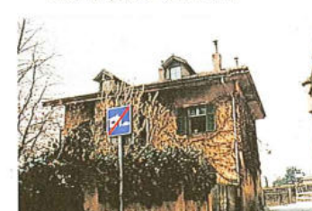
157 Casa - via Rafenstein 2 - p.ed. 138/1
