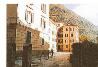
15 Palazzina - via C. Roncolo 2/4/6 - p.ed. 991
