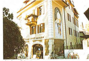
21 Casa Schrott via C. Roncolo 27b - p.ed. 26
